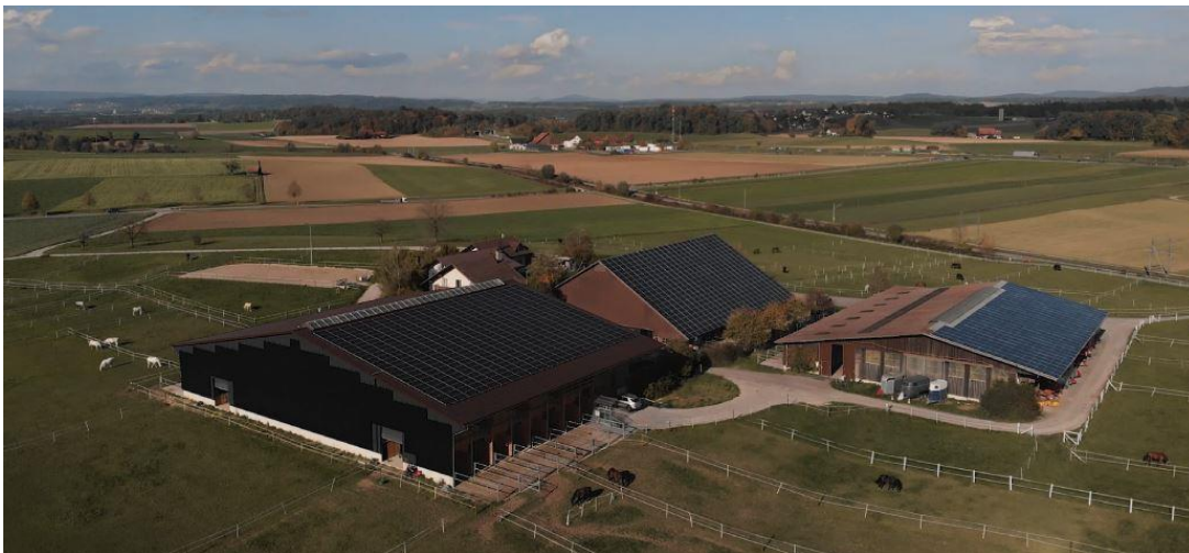
Photovoltaik-Anlage in Henggart
